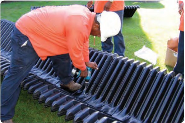
Self-tapping screws hold the channel together.
