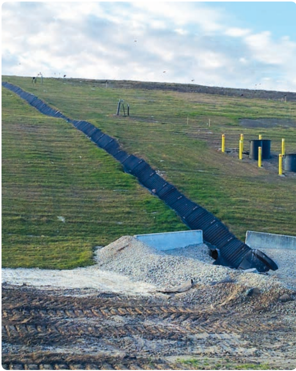
Vegetation grows up to the side of SmartDitch to minimize erosion.
