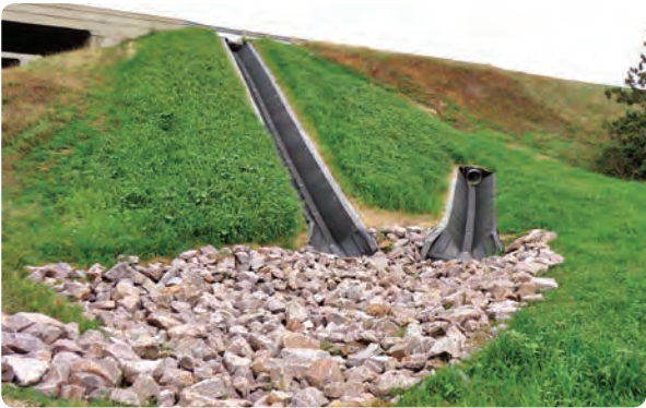
Portage, WI After: SmartDitch replaced the old Riprap, improved drainage, and eliminated erosion.
