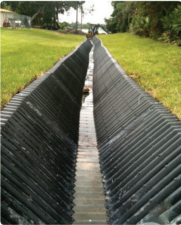
SmartDitch replaced the poor performing channel, improved flow, and required less space.
