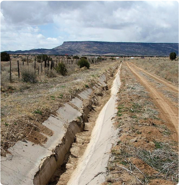
Cracked concrete irrigation ditches present major problems in rural farming communities.
