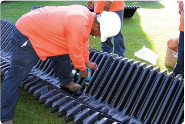
Self-tapping screws hold the channel together.
