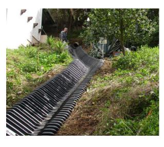
option of using SmartDitch was chosen. SmartDitch is a corrugated HDPE liner that is designed to fit into an existing or new construction ditch.
