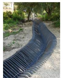
The installation of the ditch liner took approximately two days including the clearing of the vegetation and debris from the existing ditch. The installation crew consisted of local residents working with hand tools. The curves were installed by offsetting the flow line of the sections a small amount at each joint, creating a natural looking flow path. Because of SmartDitch's HDPE construction maintenance on this ditch will be minimal, ensuring years of trouble free operation.
