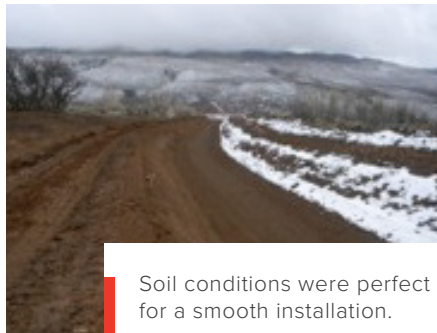
The contractor used a GPS guided blade to form the channel.
