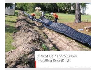
SmartDitch is manufactured in the USA. It is a safe, economical, long-lasting, and environmentally sound irrigation channel lining solution. For more information on the SmartDitch and the MegaDitch HDPE Channel Lining Systems contact:
