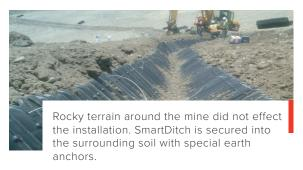
area experienced a heavy rainfall, with nearly five inches (13 cm) of rain over the course of a few hours. The SmartDitch system performed with no failures and had no significant accumulation of sediment within the channels. The SmartDitch system provided the client with a rapid, reliable and cost effective solution for stormwater run-off.
