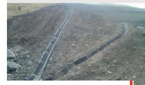
Parallel SmartDitch channels were installed to capture and carry stormwater away from the Twentymile Mine's main entrance.
