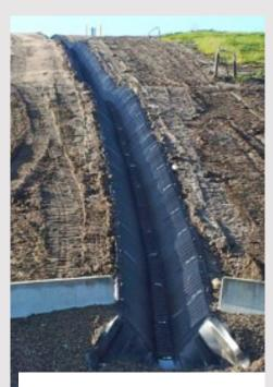
500 LF of 24" SmartDitch was installed to eliminate this landfill's perpetual slope side erosion problems, caused by large amounts of water build-up from the landfill's summit.
