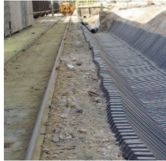
SmartDitch was the ideal channel design solution to protect the land from chemical infiltration and direct the water and chemical discharges to a containment area.
