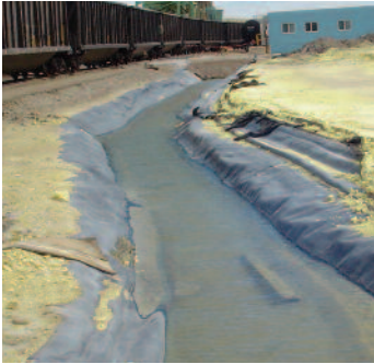
SmartDitch was the ideal channel design solution to protect the land from chemical infiltration and direct the water and chemical discharges to a containment area.
