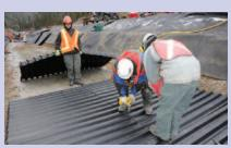
Weighing less than 75 lbs. each, the lightweight MegaDitch sections are easily moved into place.
