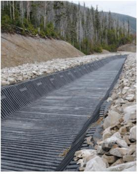
MegaDitch is made with UV resistant HDPE for excellent weatherability.
