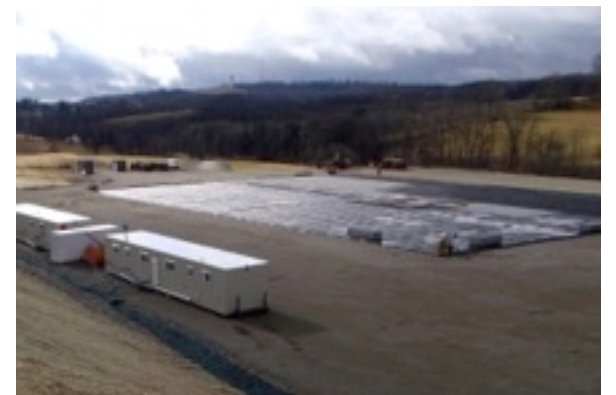
View of completed 50,000 sq. ft. lined drilling site.
