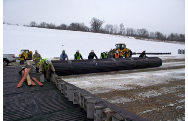
SiteSaver is unrolled into place and then electro-fused.
