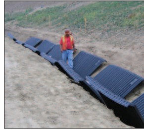
SmartDitch sections, manufactured in 8' - 10' lengths, are ready for joining in the shallow trench or above the ground and set into place.
