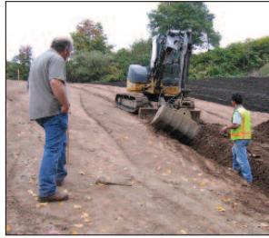
A light-duty backhoe is all that is needed to dig the shallow trench in preparation for the SmartDitch installation.
