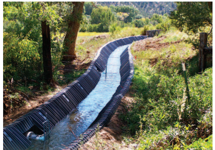
Many irrigation ditches, canals and laterals run through uneven terrain and difficult-to-access areas.
