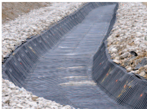
No sandblasting or special equipment is required for SmartDitch MegaDitch installation. See the MegaDitch brochure for installation instructions.
